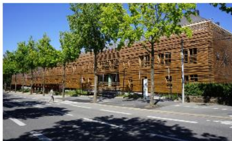
Centre de formation Copernic - Angers (49)
