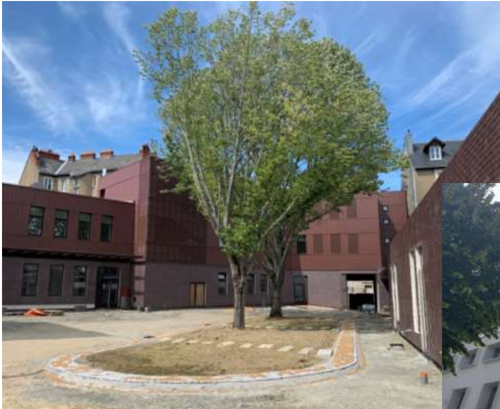
Futur collège Nantes Centre (ex-lycée Vial) NANTES
